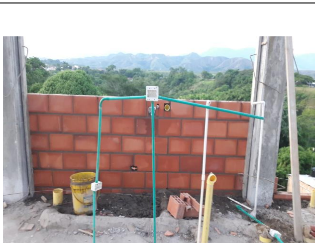
Instalacion tuberia electrica torre B
