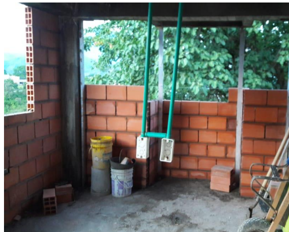
Instalacion tuberia electrica torre a
